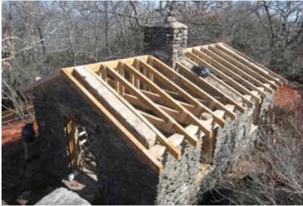
Beams & rafters, hauled by pack team, installed, ready for shingles
